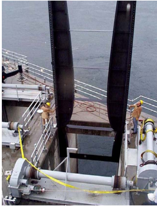
Figure 1: Variable-width, fixed shape salmon ladder Entrance Weir at Wanapum Dam
